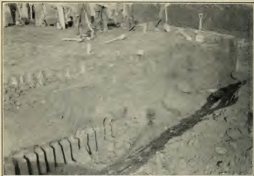
a. Vertical cleavage plane between earth inside structure and outside structure. Outside has split off nearly up to shovel standing vertically. Mound No. 1, Site No. 2.
