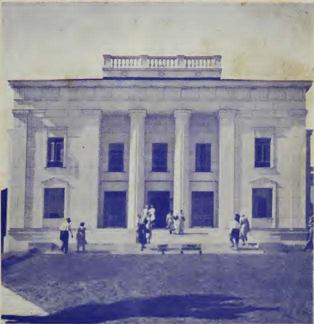
Pioneer Memorial Building
